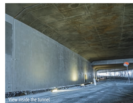
View inside the tunnel
