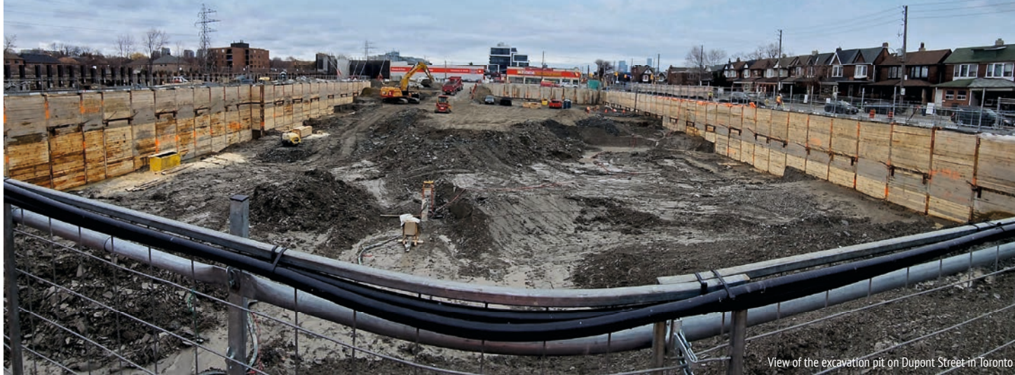
View of the excavation pit on Dupont Street in Toronto
