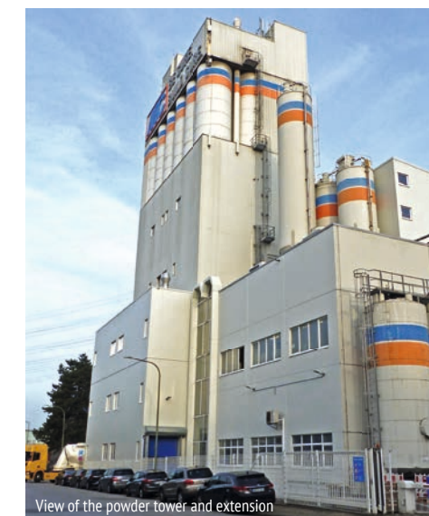
View of the powder tower and extension
