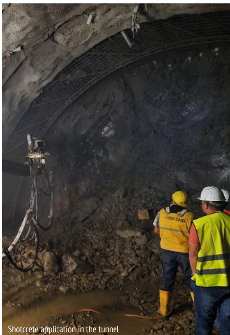
Shotcrete application in the tunnel
